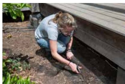
Subfloor Application demonstrating no specialty tools are required, scissors and staple gun were used Bushfire Mesh FLEXI Shield
