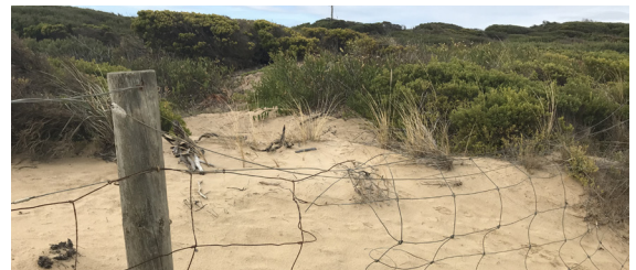
Figure B Galvanised fencing materials cannot withstand Australia's harsh coastal environments.
