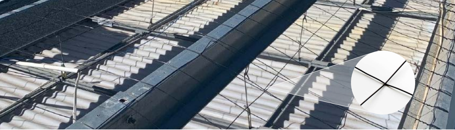
Figure C Roof Safety Mesh installation in progress Photo Credit: Murphy's Remedial Builders
